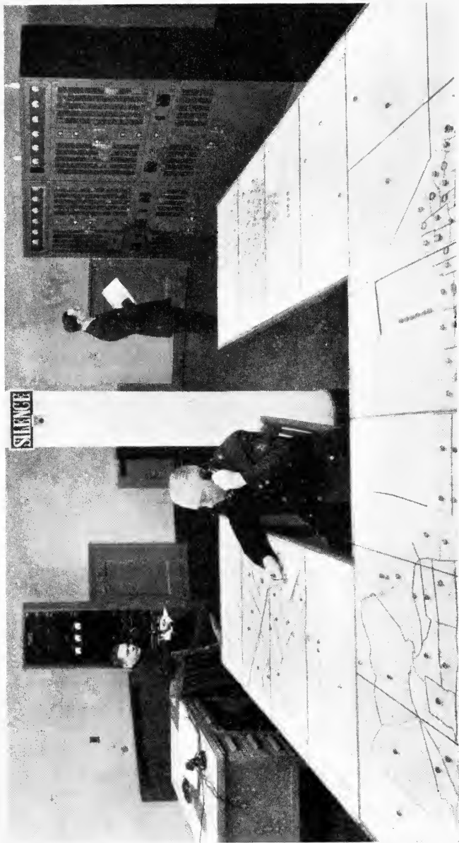
The nerve center of the New York City police radio patrol system. The dispatcher is surrounded by maps of the city's boroughs which indicate by metal disks the location of all patrol cars on duty. Note, in background, transmitter at right, speech-input system at left.
